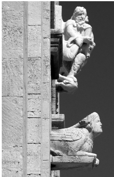
Figure 8: The Sphynx in the Southern Façade of the Trani Cathedral
